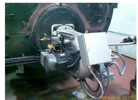
Above: The Riello Burner fitted with Autoflame components
