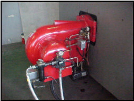
Autoflame fuel and air servos.
