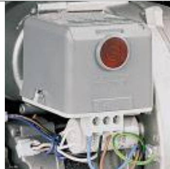
Control box fitted with an ignition transformer
