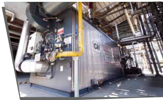
Multitubular heaters for medium to large capacity
