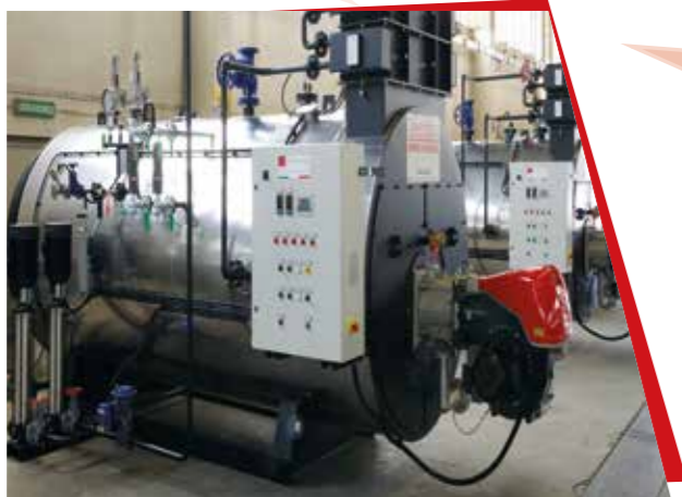
Fire tube steam generators, small to medium capacity
