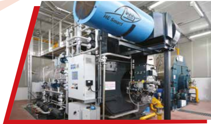
Fire tube steam generators medium to large capacity, efficiency up to 97,5%
