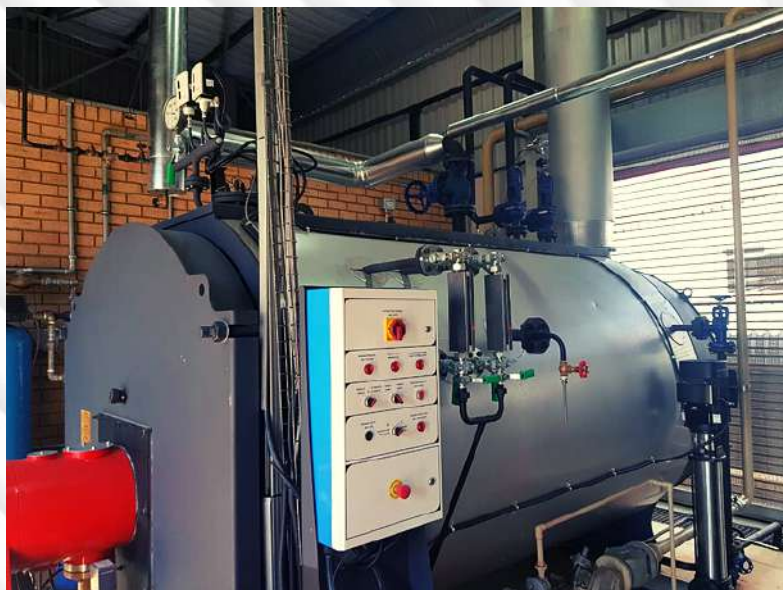
24/7 Combustion Technology Boiler Management System Interface
