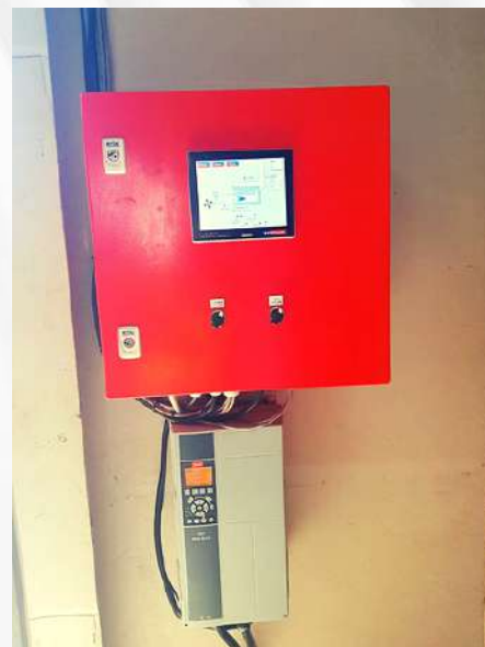
24/7 Combustion Technology Boiler Management System Interface
